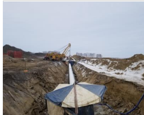
Description & Location KP-826+700
