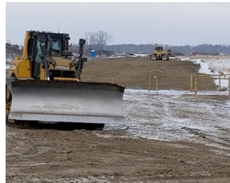
Description & Location KP-842+883
