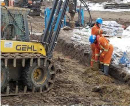
Description & Location KP-819+100
