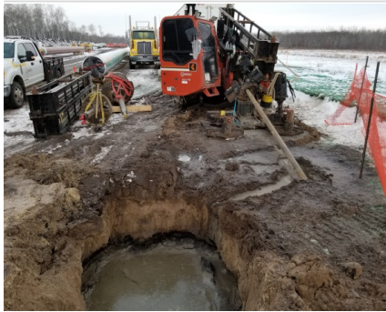
Description & Location KP-863+300
