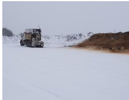
Description & Location KP-813+200
