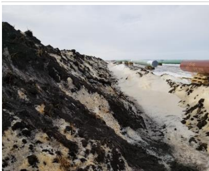
Description & Location KP-903+400
